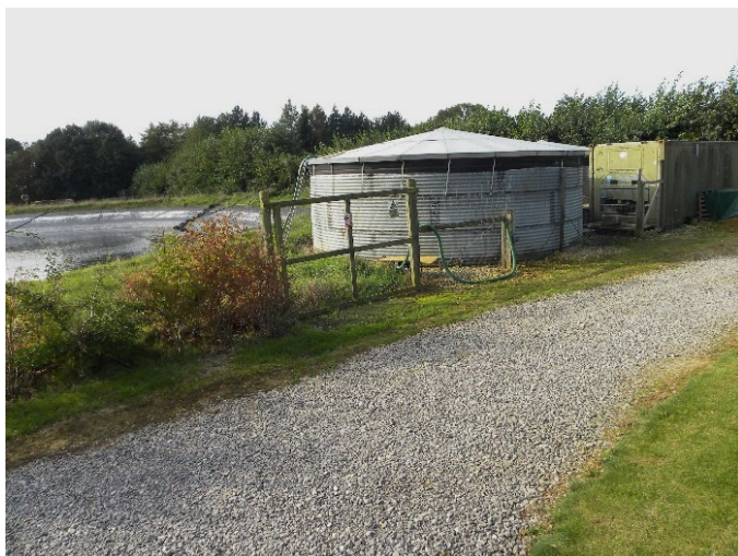
Above left – water treatment and storage at Nicholsons. Water is drawn from the main reservoir, treated and then stored in covered water tanks to minimise the risk of contamination with Phytophthora species. Above right – waste management at Nicholsons. All waste materials are carefully sorted and stored so that each waste material type can be treated and disposed of appropriately or safely used, e.g. for sustainable energy generation.
