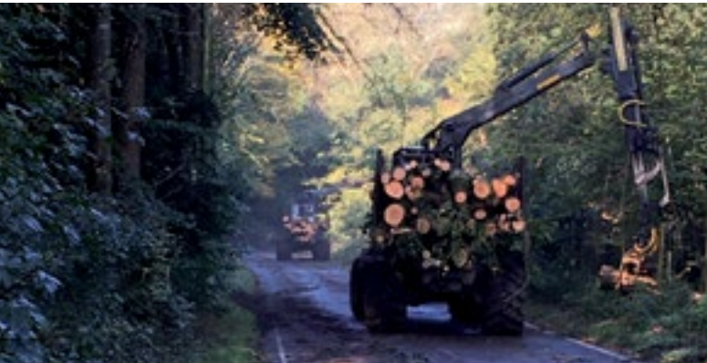
Forwarders at work on the B2141
